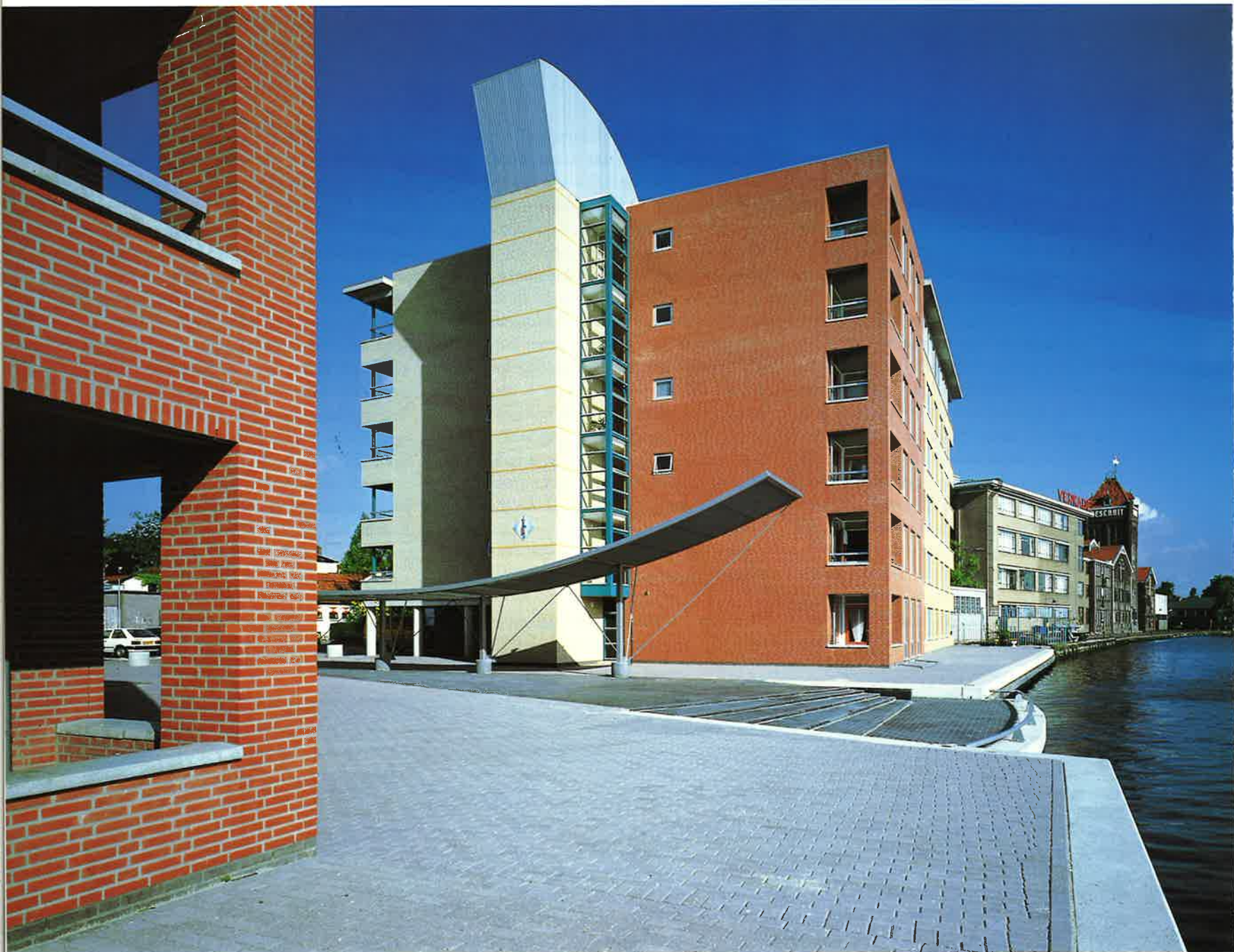
Woningbouwproject in Zaandam, Pieter Wester (Inbo/Gjalt de Jong)
